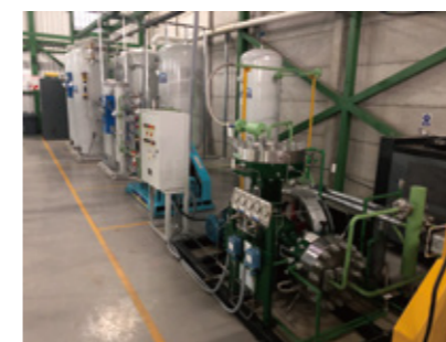
Peru Hospital geriatrico Cerro Colorado
